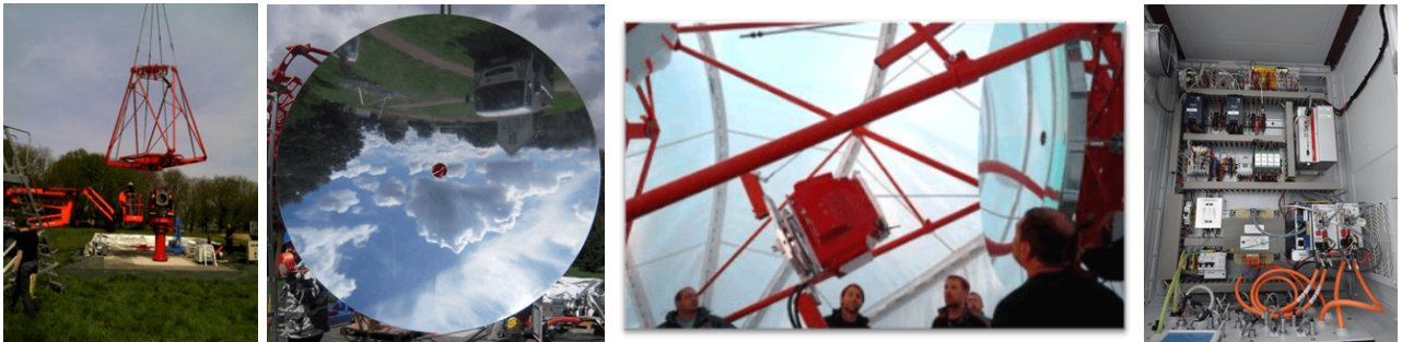
Fig. 5. Integration of the complete prototype. From left to right: (I) mounting the OSS on the tower and the AAS in April 2015, (II) the secondary mirror during its installation on the mechanical structure in August 2015, (III) first loading of the camera on the telescope in November 2015, (IV) the main cabinet for the slow control of the instrument.
