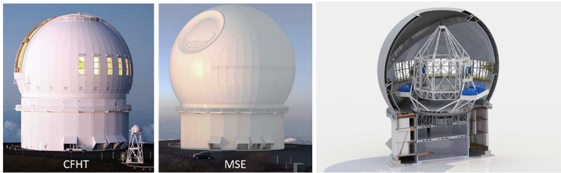
Fig. 1. Left: View of the present CFHT. Middle: View of the studied MSE with a 10 percent larger than the CFHT modern calotte enclosure. Right: MSE Conceptual System Design Configuration Overview.
